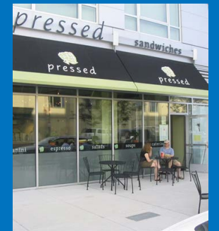
Non-retractable, Fabric Awning Sign with Non-Illuminated, Printed Business Name on Awning Main Cover
