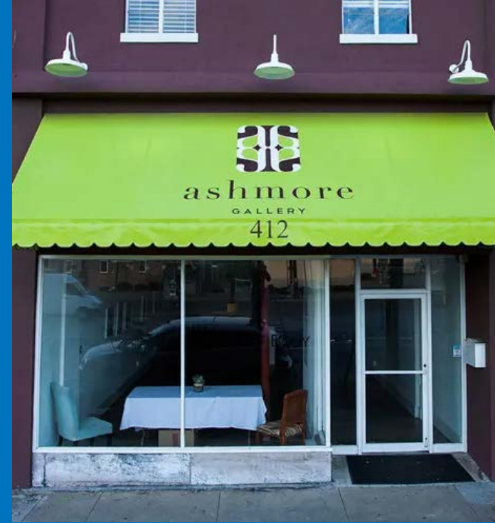
Non-retractable, Fabric Awning Sign with Externally-Illuminated, Screen-Printed Business Name on Awning Main Cover and Valance
