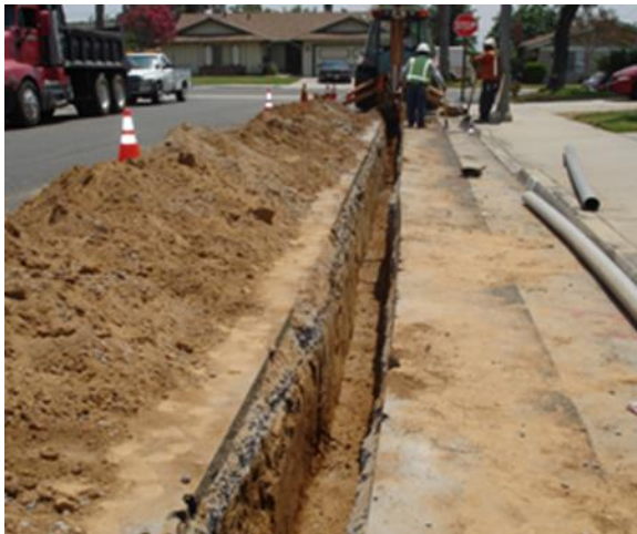
Trench and Conduit Installation
