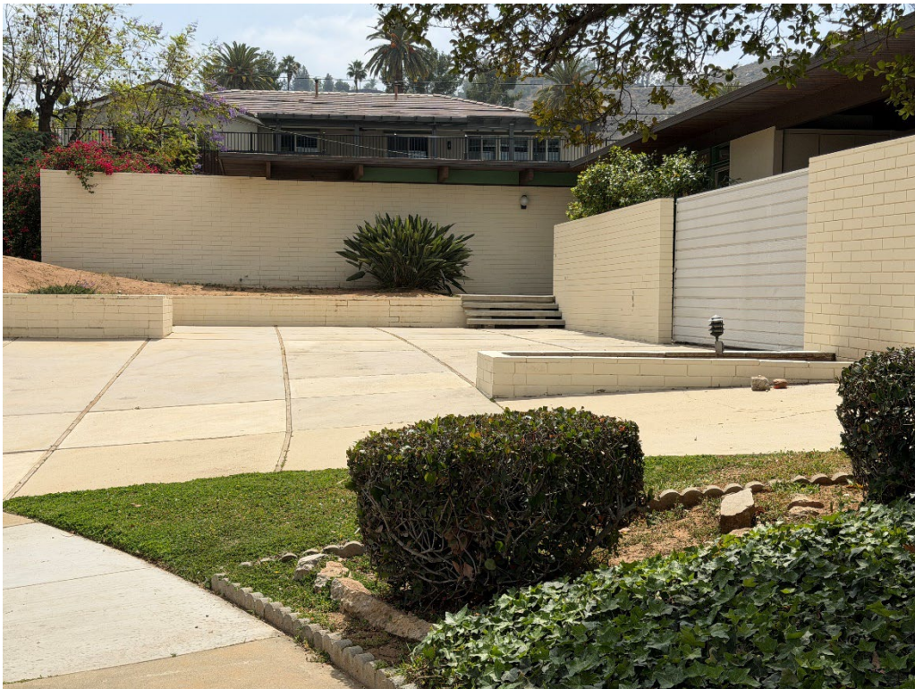
Figure 2 – Edie façade, secondary front elevation, and driveway, view east/southeast
