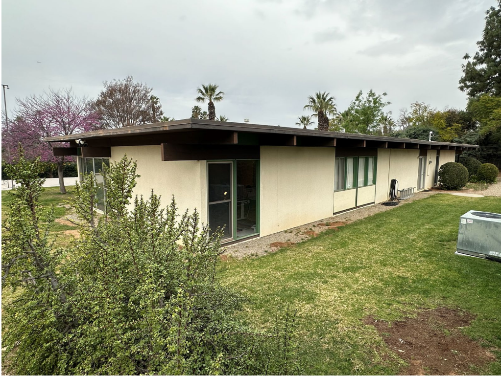
Figure 9 – Rear and east side/rear elevation showing example of double-hung vinyl replacement of jalousie window in original opening, view northwest
