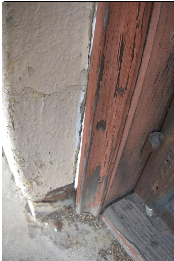
Barley Mills Building Exterior Window wood trim: Source G T Louden AIA Photography, November 2103; Detail of window jamb, plaster veneered brick recess and sill. Figure # D-22
