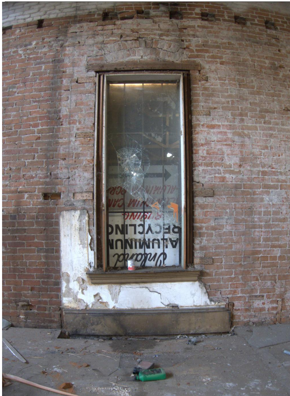
Barley Mills Building Interior : Source G T Louden AIA Photography, November 2103; Detail of window jamb, sill, apron trim weight box and plaster veneered brick recess at base trim. Figure # D-23
