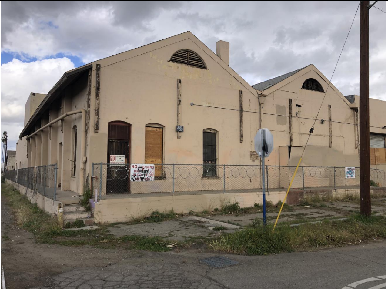
Figure # 22: Existing site context, photograph dated 2022; south façade of the Barley Mills Building and the original wood framing supports for the original canopy at south gable and at west façade. Existing chimney at southeast gable is not visible in the 1906 era photograph. This chimney is not proposed for retention without structural retrofitting.
