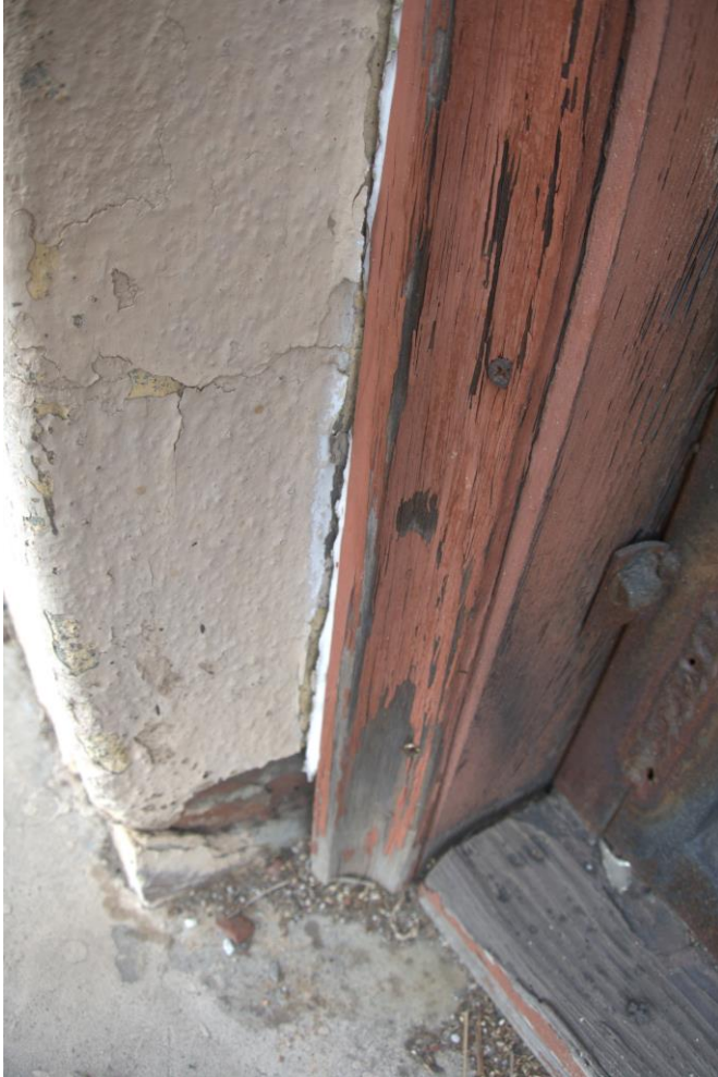
Barley Mills Building Exterior Window wood trim: Source G T Loudon AIA Photography, November 2103; Detail of window jamb, plaster veneered brick recess and sill. Figure # D-22
