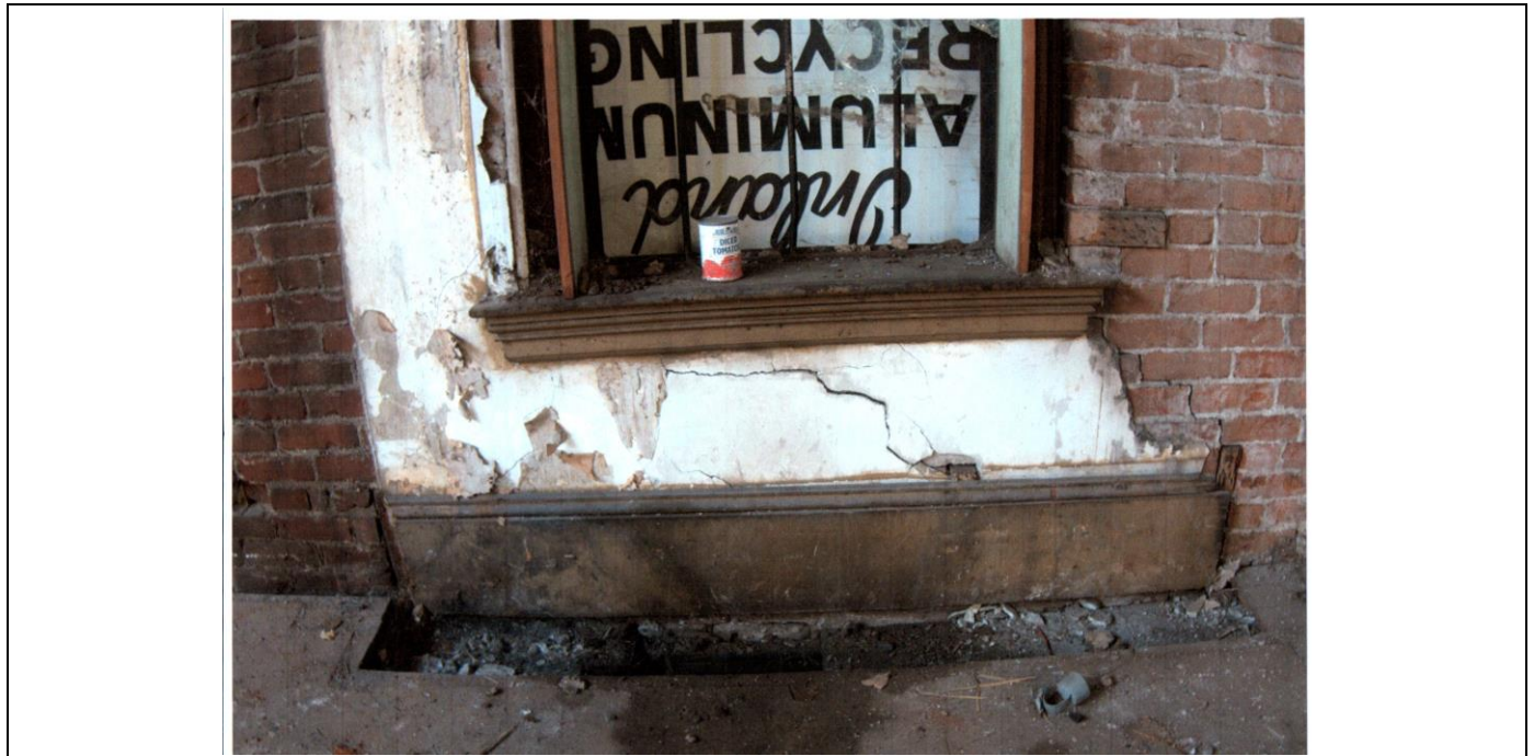
Figure # 20: The remaining original south façade interior wood window trim details at the named "office" area of the Barley Mills Structure: wall base and trim cap; window apron, window sill, window jamb trim/sash window weight box. See Appendix D.
