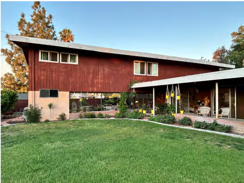
Figure 6 - West elevation, view looking northeast
