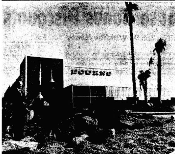
Bourns, Inc. Headquarters (1960-1964)
