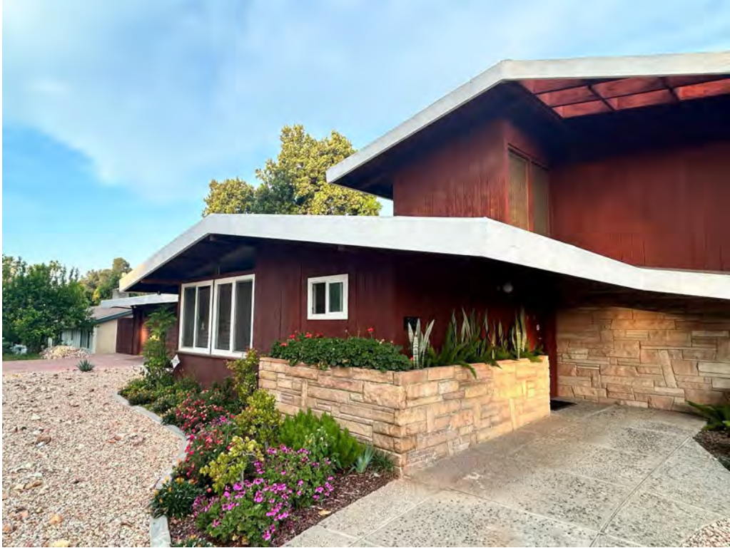
Figure 5 - Main entry, view looking west
