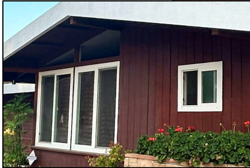
Examples of window replacement
