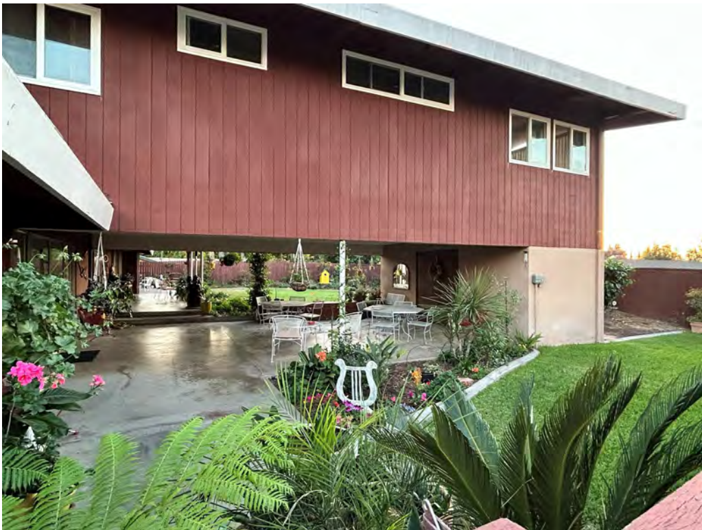
Figure 8 - East elevation, view looking west
