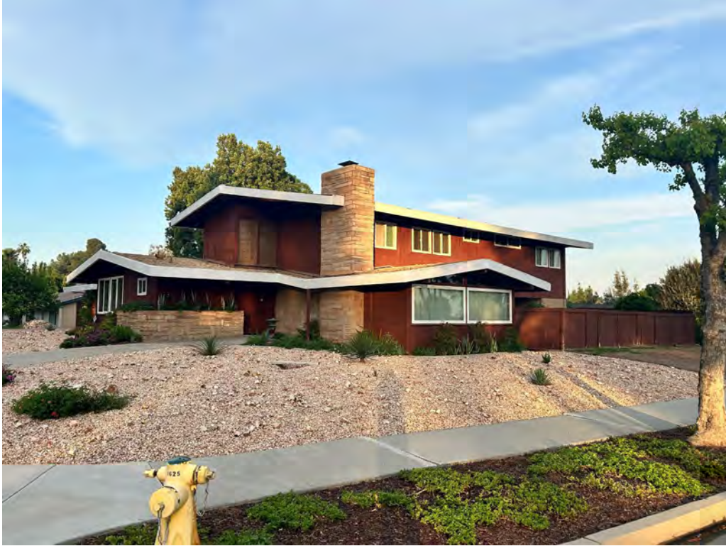
Figure 3 - Secondary (east) facade, view looking west
