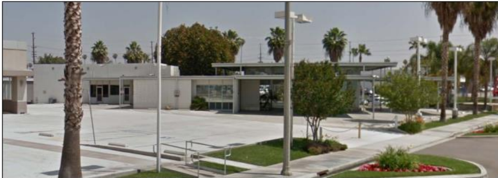
Southwest elevation. Original building configuration prior to demolition of the southern block of the building in 2012.
