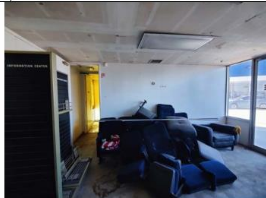
Rear of building (northwest area), office space.
