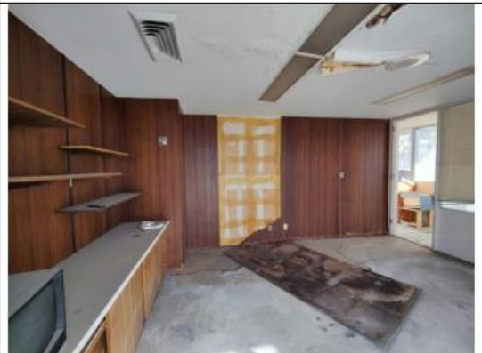
Rear of building (northwest area), office space.
