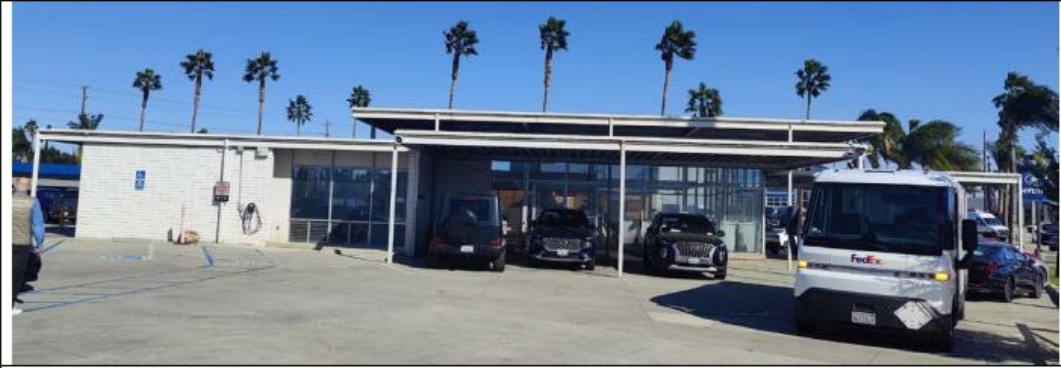
Southern elevation, facing northeast.
