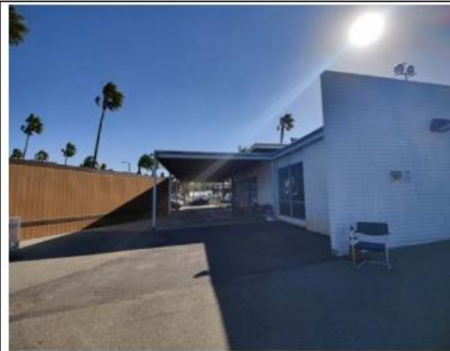
Northeast elevation, facing southeast.
