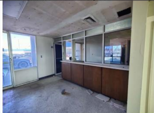
Rear of building (northwest area), office space.
