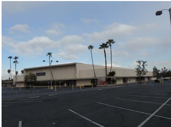
View of the East Façade, looking Northwest (February 2013)
