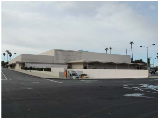
View of the North Façade, looking Southwest (February 2013)
