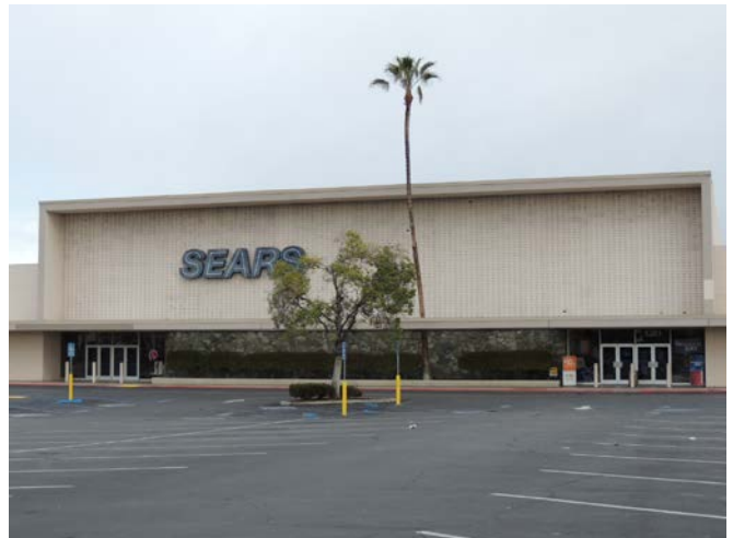
Detail of South Façade (February 2013)
