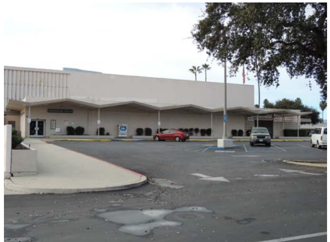
Detail of the Folded Plate Roof (February 2013)
