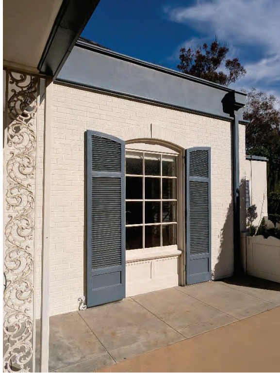
Figure 7 - Example of segmented arch topped window openings and tall/narrow shutters
