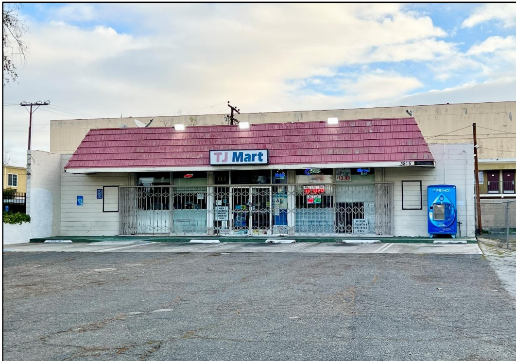
Existing TJ Mart convenience store to be demolished
