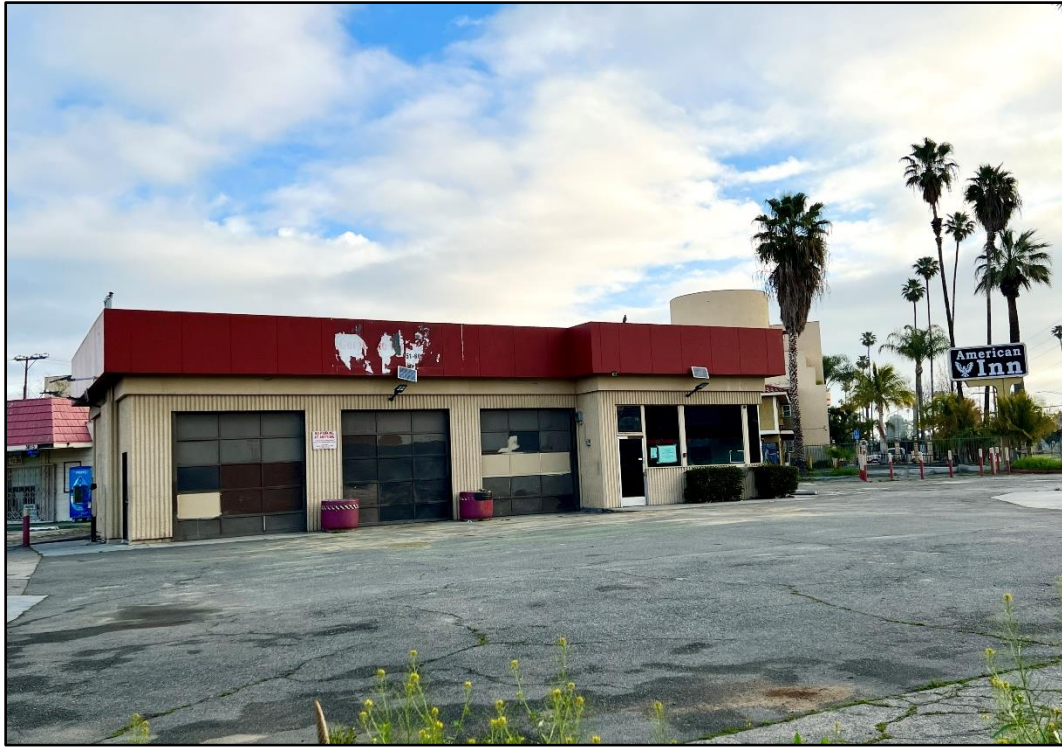
Existing vacant vehicle repair facility to be demolished
