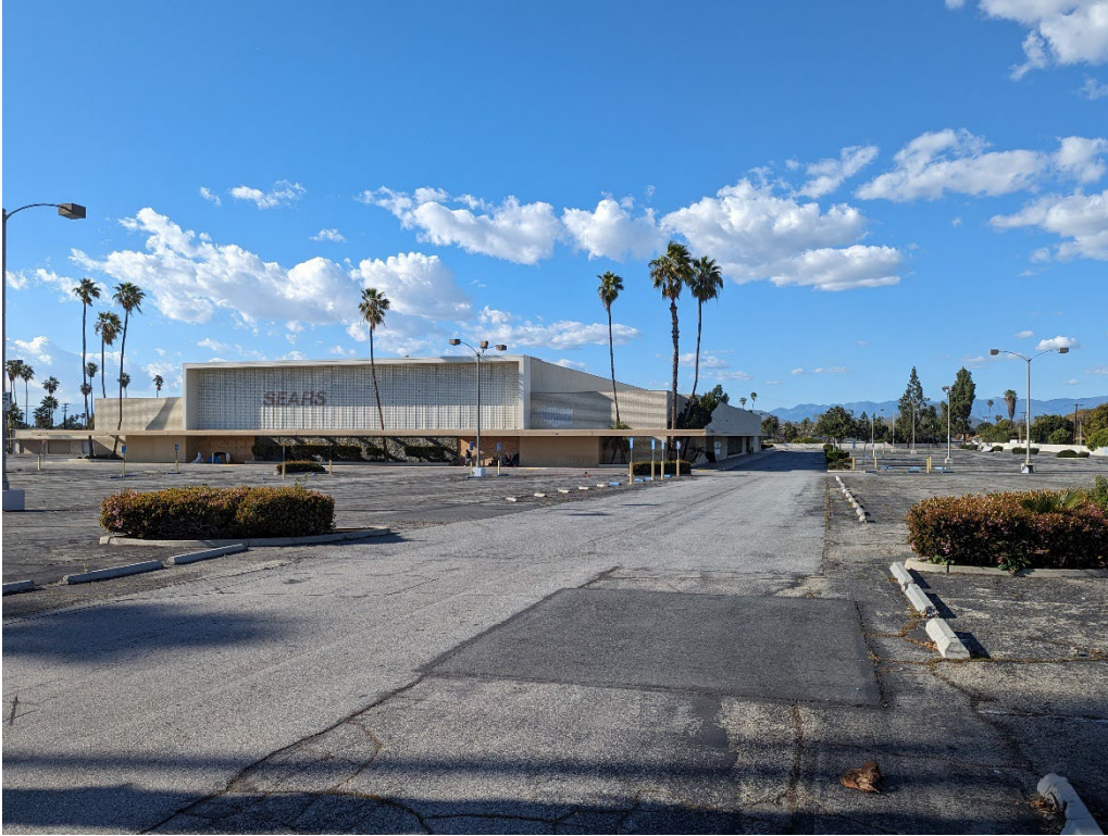
Figure 1 - View from Arlington Avenue
