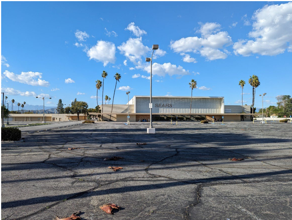
Figure 8 - South (Front) Elevation, from Arlington Avenue
