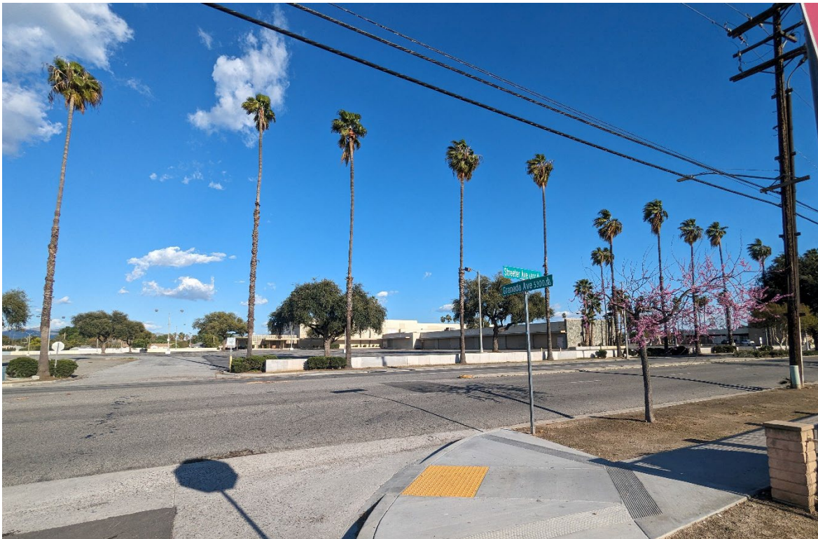
Figure 10 - Rear view from across Streeter Avenue
