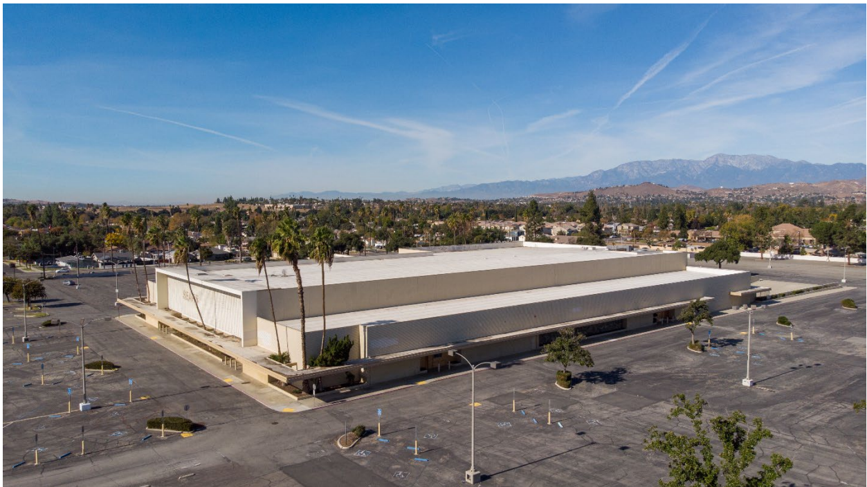
Figure 12 - Bird's eye view looking northwest
