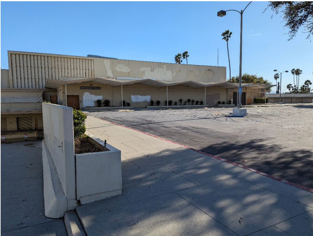
Figure 4 - North (Rear) Elevation
