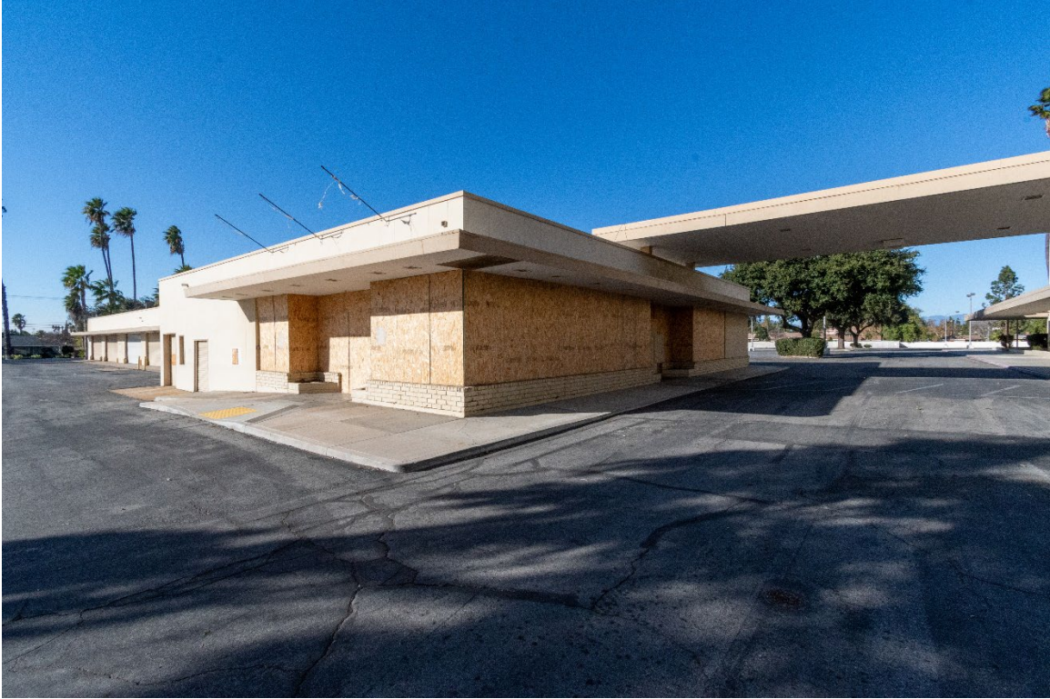
Figure 7 - Auto Service Center
