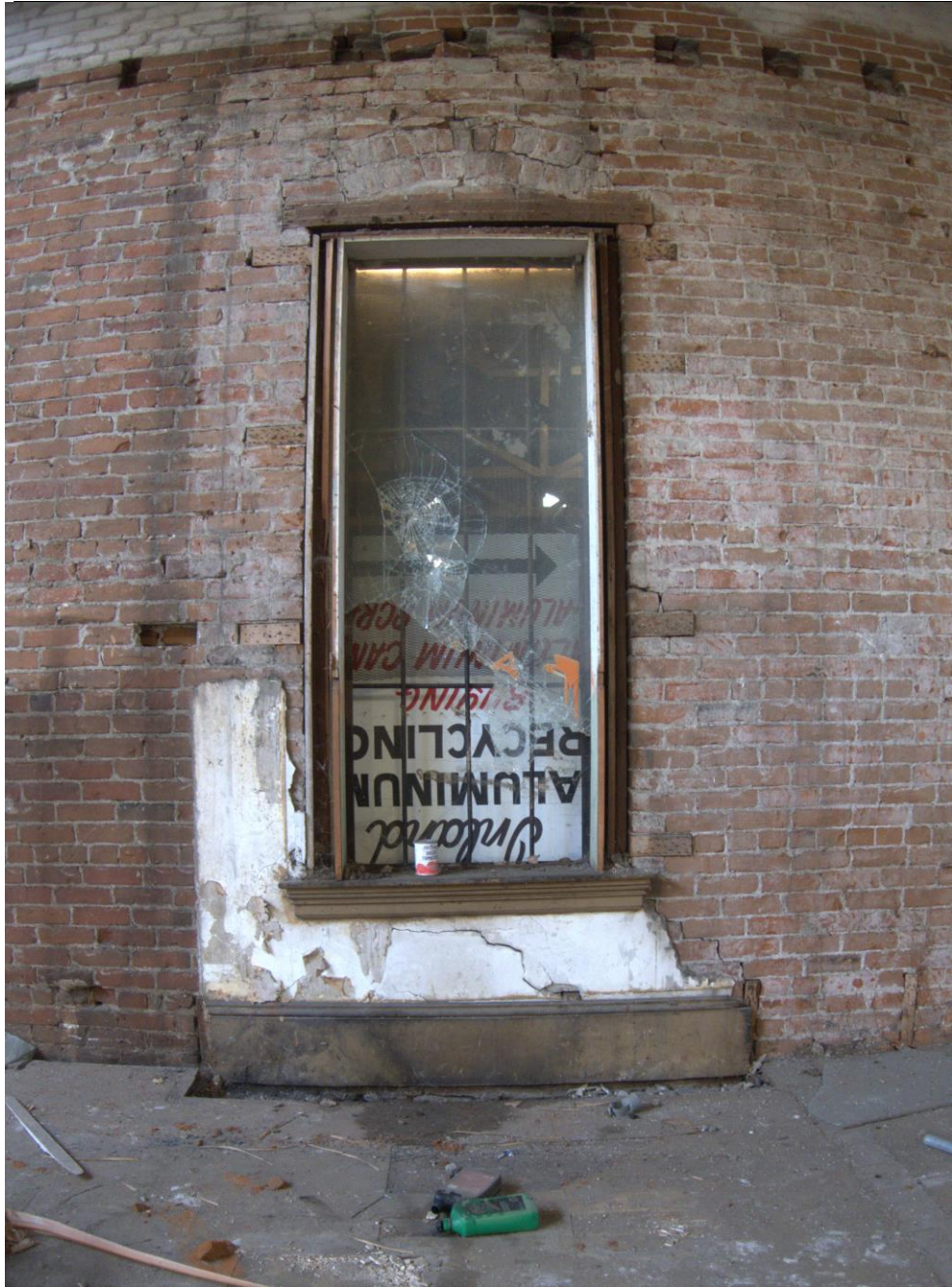
Barley Mills Building Interior : Source G T Loudon AIA Photography, November 2103; Detail of window jamb, sill, apron trim weight box and plaster veneered brick recess at base trim. Figure # D-23
