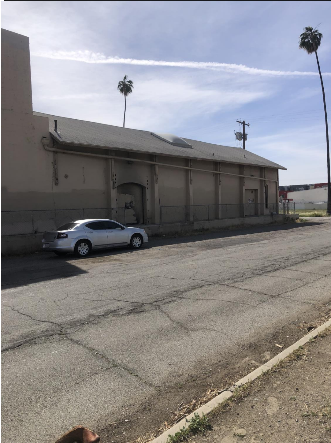
Barley Mills Building Exterior: Source G T Louden AIA Photography, March 2022; Overview of west façade; the taller mass at the left side is part of the 1930 era addition; skylights are not original and are not proposed to be restored. Figure # D-19
