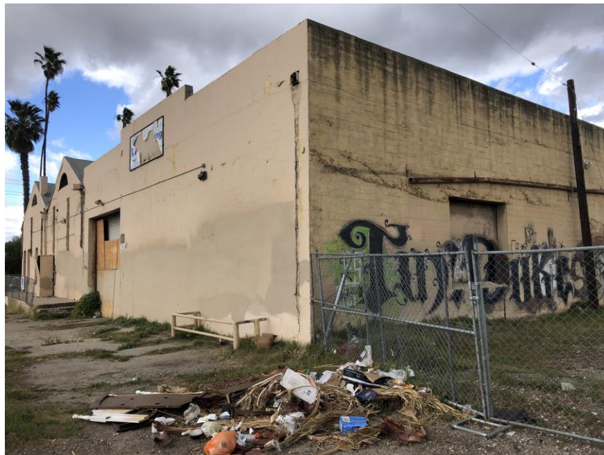
Figure # 21: Existing site context, photograph dated 2013; Barley Mills Building twin gables at the south elevation. The 1930 concrete wall addition is in foreground of the southeast corner.
