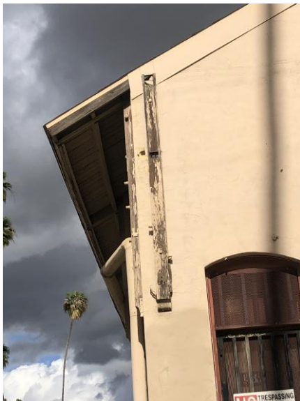
Barley Mills Building: Source G T Louden AIA Photography, February 2022; Portion of South façade showing wood frame bolting to the URM wall, supporting non-extant canopy; note the projecting roof overhang that conceals the original continuous roof vent; Figure D-12
