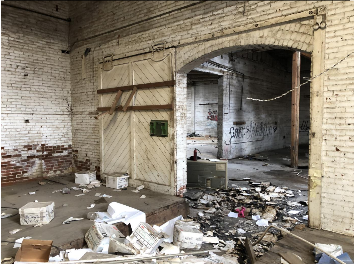
Barley Mills Building Interior: Source G T Loudon AIA Photography, February 2022; Figure # D-15 View to east of original triple wythe segmented brick arch opening in original east exterior façade. View through opening is of the concrete walls structure of the later 1930 additions.
