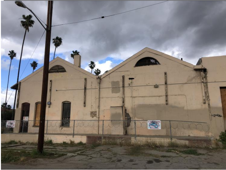
Barley Mills Building, South façade double gable detail.
