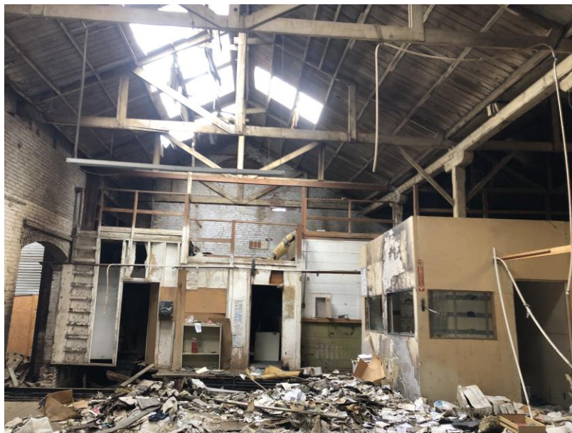
Figure # 19: Interior photographs, 2022 showing non-contributing interior build-out construction prior to their removal. The remains are clear expressions of the spatial volume with trusses, exposed brick walls, and triple- segmented arched masonry doorway openings. Raised wood flooring visible in the foreground is severely damaged by fire at the southeast corner.
