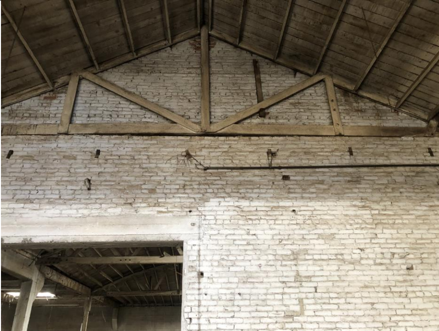
Barley Mills Building Interior: Source G T Loudon AIA Photography, March 2022; Overview of north façade; note the truss members are slightly recessed in the brick wall. Note the opening with a steel head lintel, indicating this was a newly creating opening. Figure # D-20
