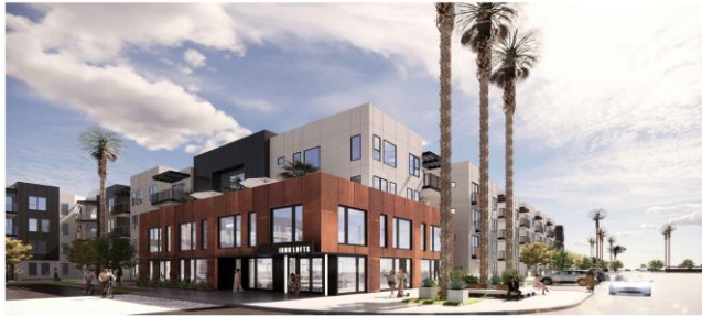
LEASING LOBBY PROJECT ARRIVAL | BUILDING A
