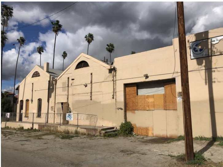
Barley Mills Building: South façade, doubled gable. Parapet to the east is the 1930 concrete addition.
