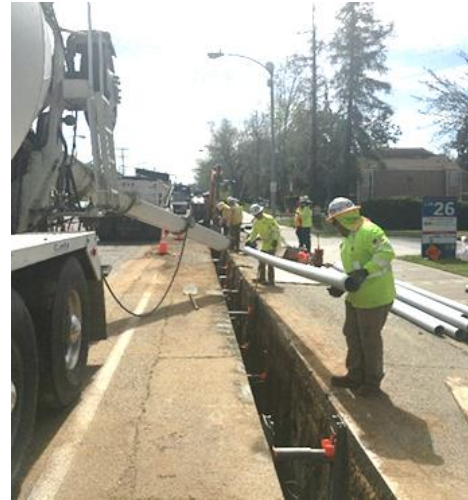
Typical Trench and Conduit Installations
