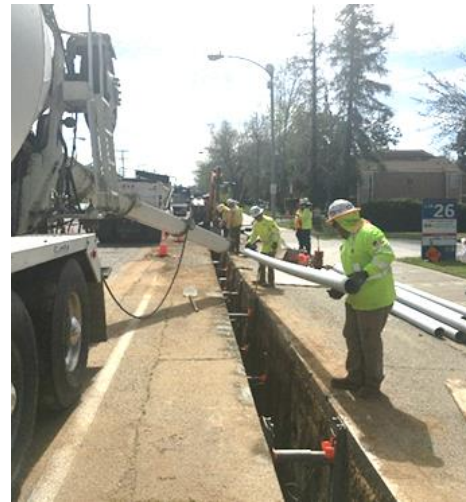
Typical Trench and Conduit Installations
