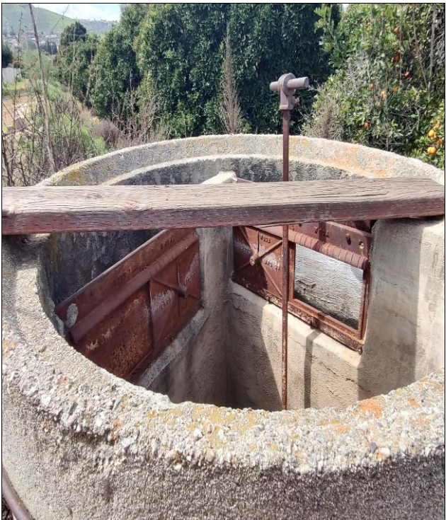
Figure 6. Master valve at the eastern end of Site 33-023901. (Photograph taken on March 13, 2024; view to the west)
