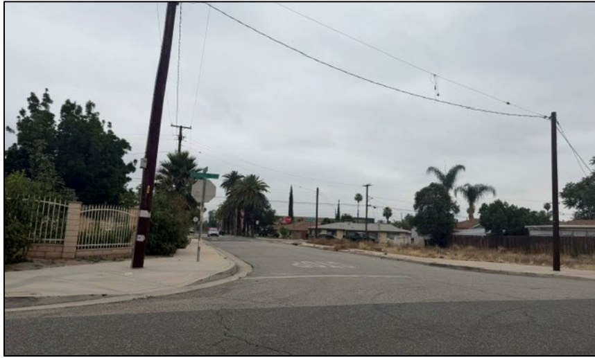
Winstrom Street; between Casa Banca Street and Railroad Avenue
