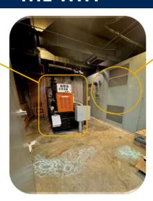
1960s era main switch gear is producing decibel levels of 90-100 (this is between levels for a gas lawn mower and motorcycle).
