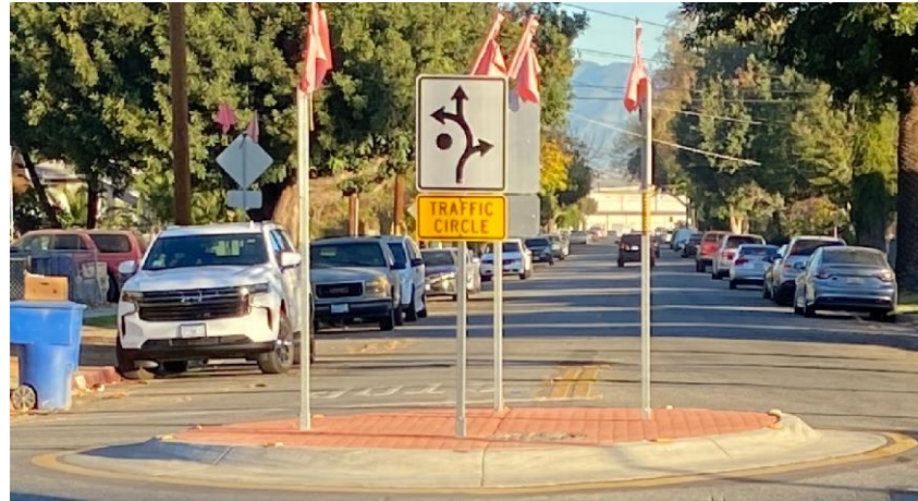
Neighborhood Traffic Circle
