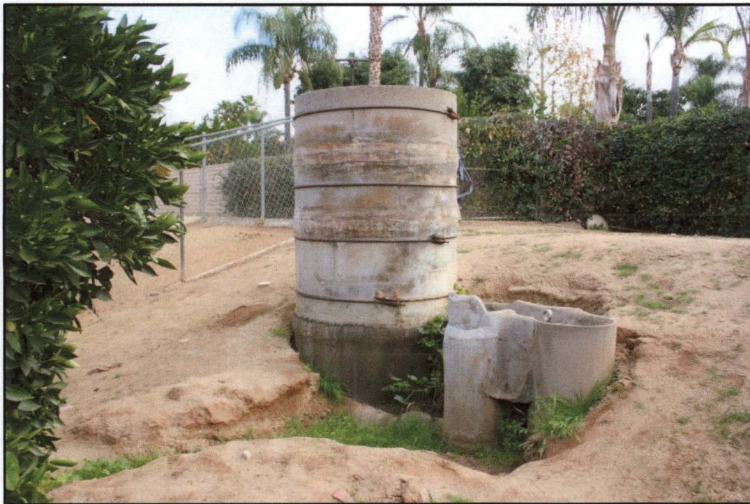
Large standpipe irrigation feature in eastern corner of the property (East)
