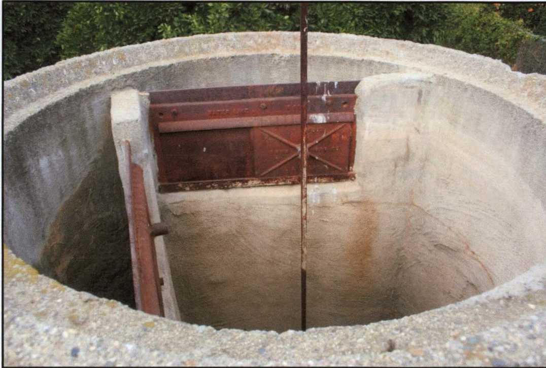
Interior of large standpipe feature (see previous photo; Close-up)
