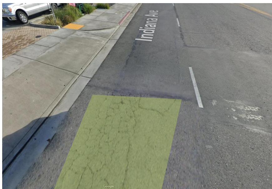
Figure 5. Propagating Cracks (Highlighted) Near Patch on Indiana Avenue
