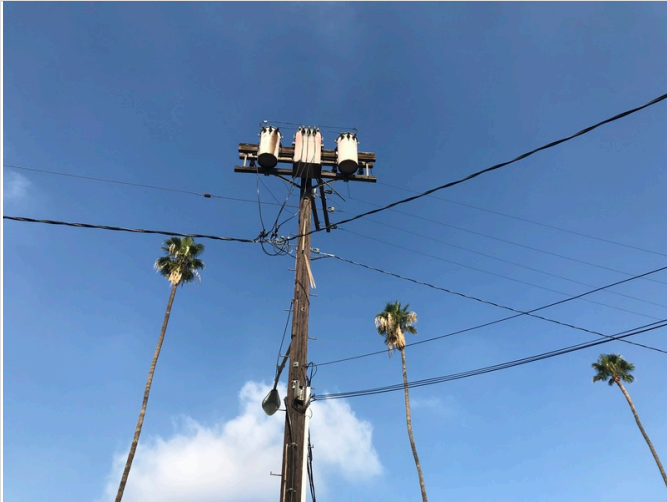
31. Pole-mounted transformers
