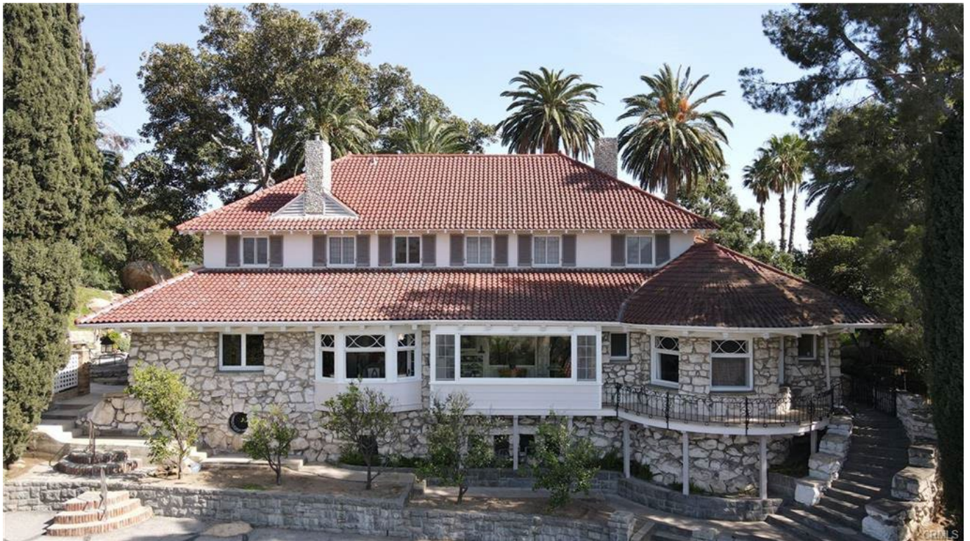
Figure 10 - Rear elevation, view looking southeast
