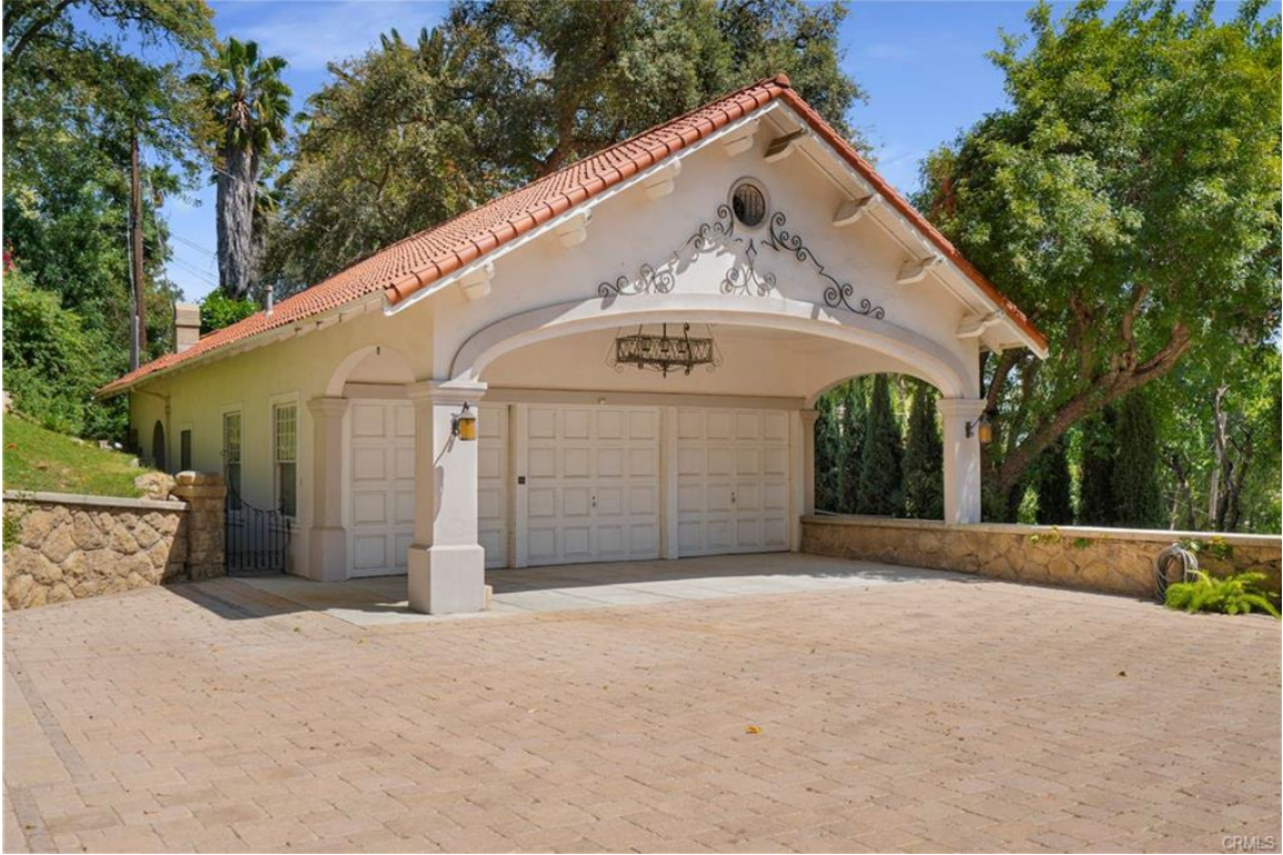
Figure 19 - Garage, view looking west
