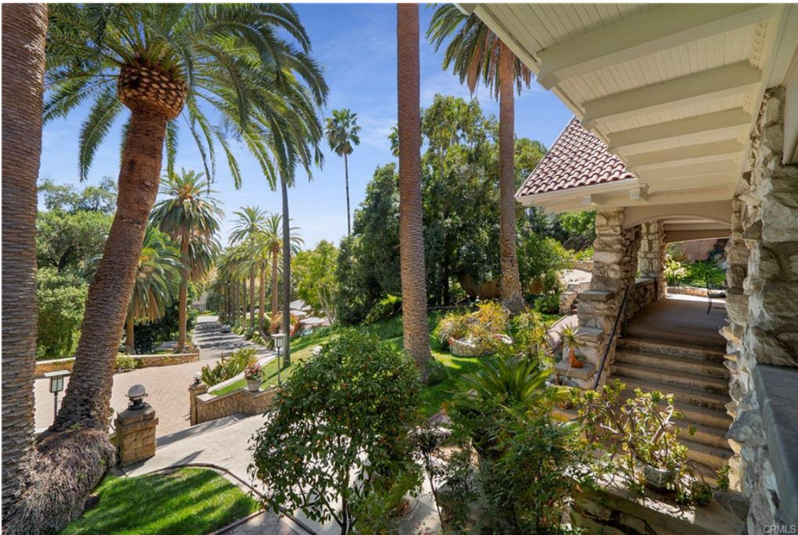
Figure 6 - Front porch, view looking southwest
