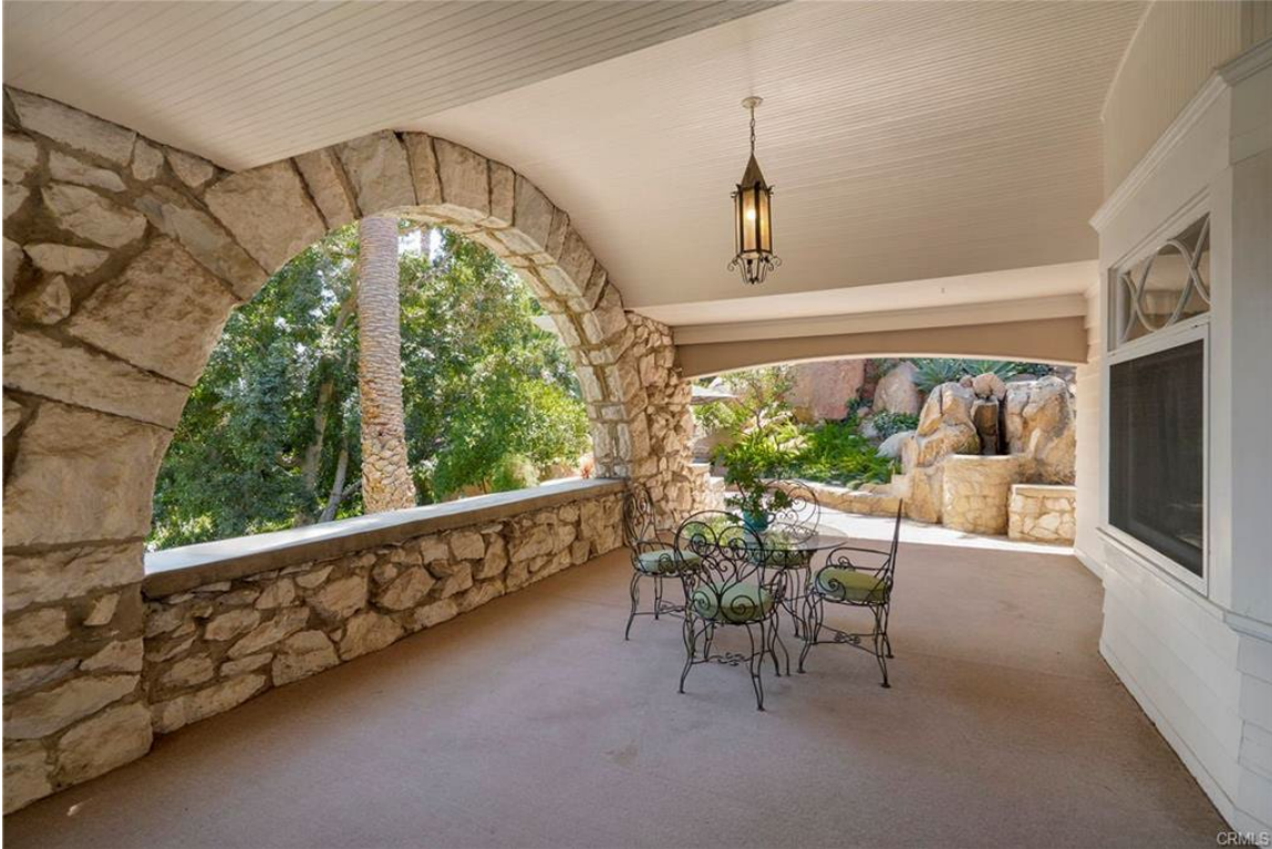
Figure 7 - Front porch, view looking southwest
