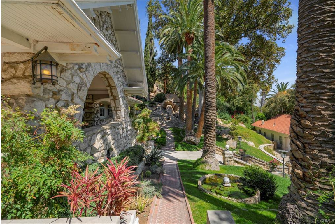
Figure 5 - Front porch, view looking northeast
