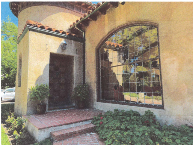
Entry and fenestration detail, view N/NE
