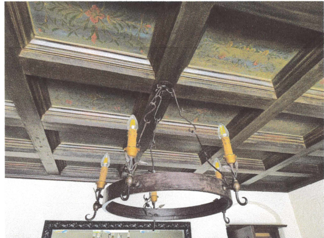
Interior dining room original ceiling and light fixture, view N
