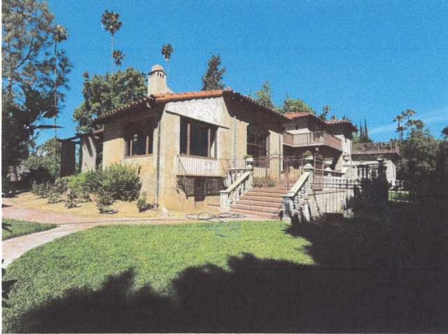
Original southerly side and rear elevation, view NW
