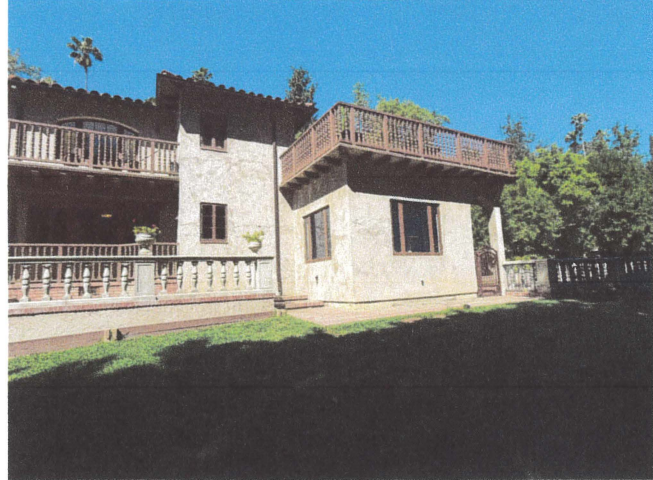
Elevator and Gym with Deck Addition (2010), view NW
