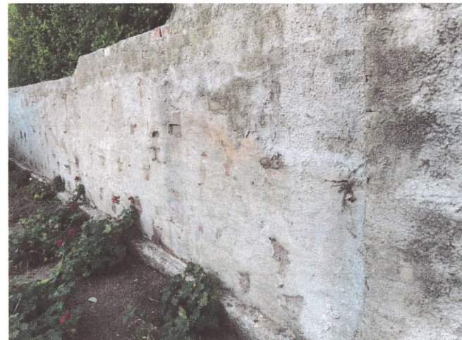
Front perimeter wall detail (1890s-1904), view SW
