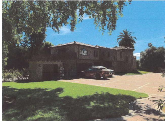
Northerly side elevation and façade, view SE
