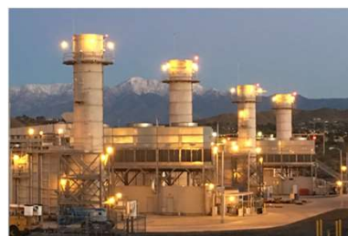
Riverside Energy Resource Center (RERC) (196 MW)
