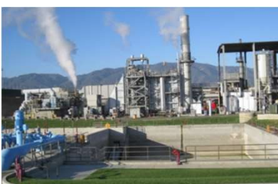
Clearwater Power Plant (28MW)
