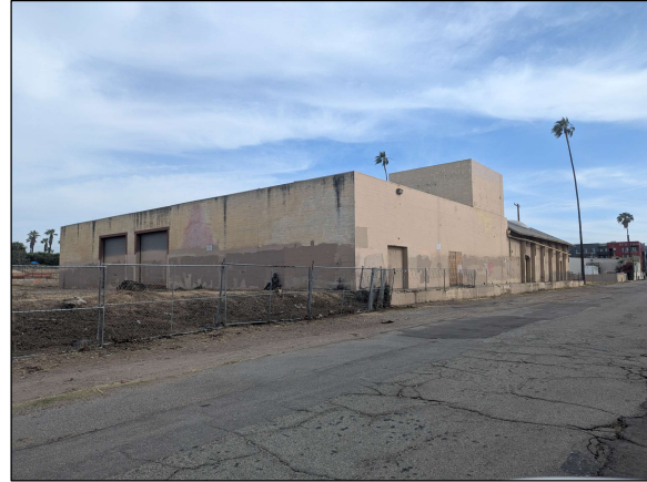
Non-original addition, looking southeast
