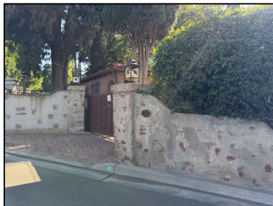
Perimeter wall and gate house
