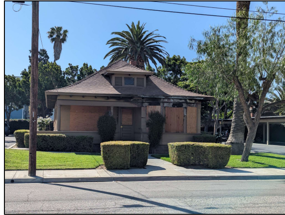
Demolished Structure at 4472 Orange St
