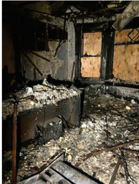
Photo 8. Office with bay window (2024).
