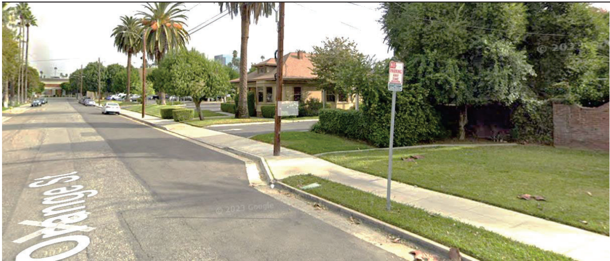
Photo 1. Streetscape. The streetscape transitions from a residence (out of view far right side of the photo) in the PPHD, to covered parking (obscured by shrubs), to the residence converted to an office (4472 Orange Street, middle of the photo), to a parking lot and commercial uses further north. Source: Google (2023).
