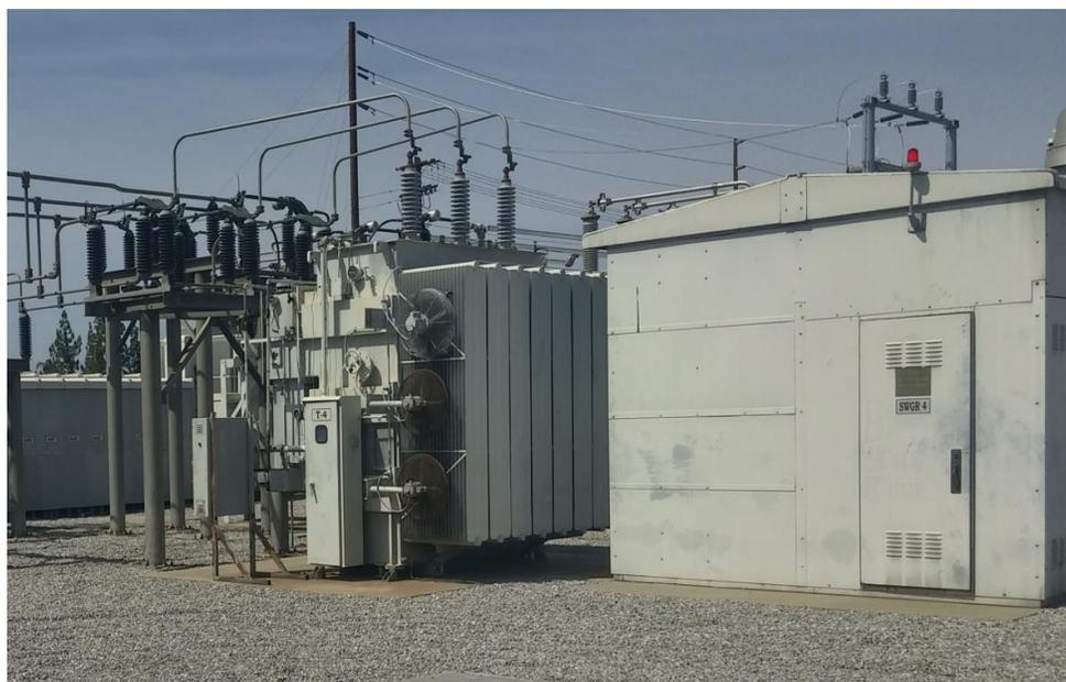
*Switchgear No. 4 and Transformer T4 to be removed at Plaza Substation*
