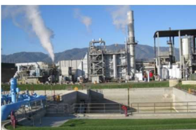
Clearwater Power Plant (28MW)
