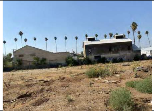
View of the Property from the southern corner
