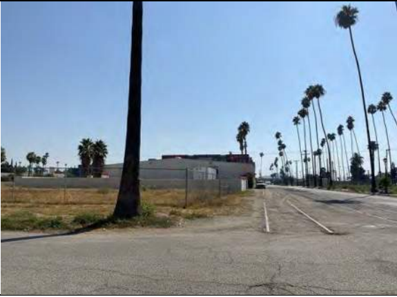
View of former rail road spurs along Commerce Street
