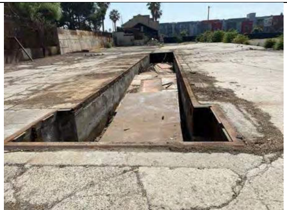
View of concrete pits - former scale with metal plates
