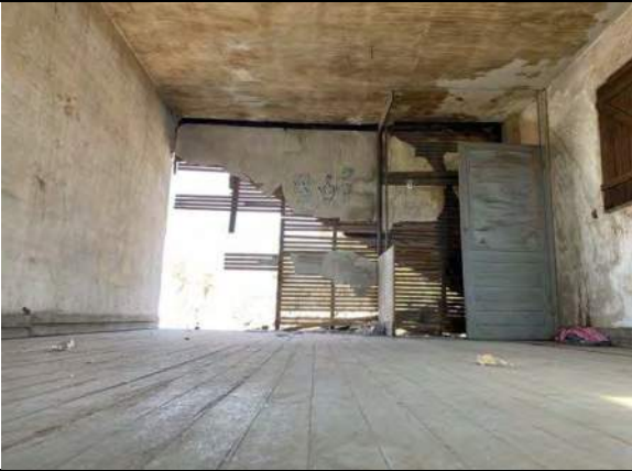
Interior view of the building on southeast portion of the Property
