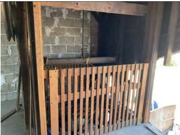
View of former elevator shaft
