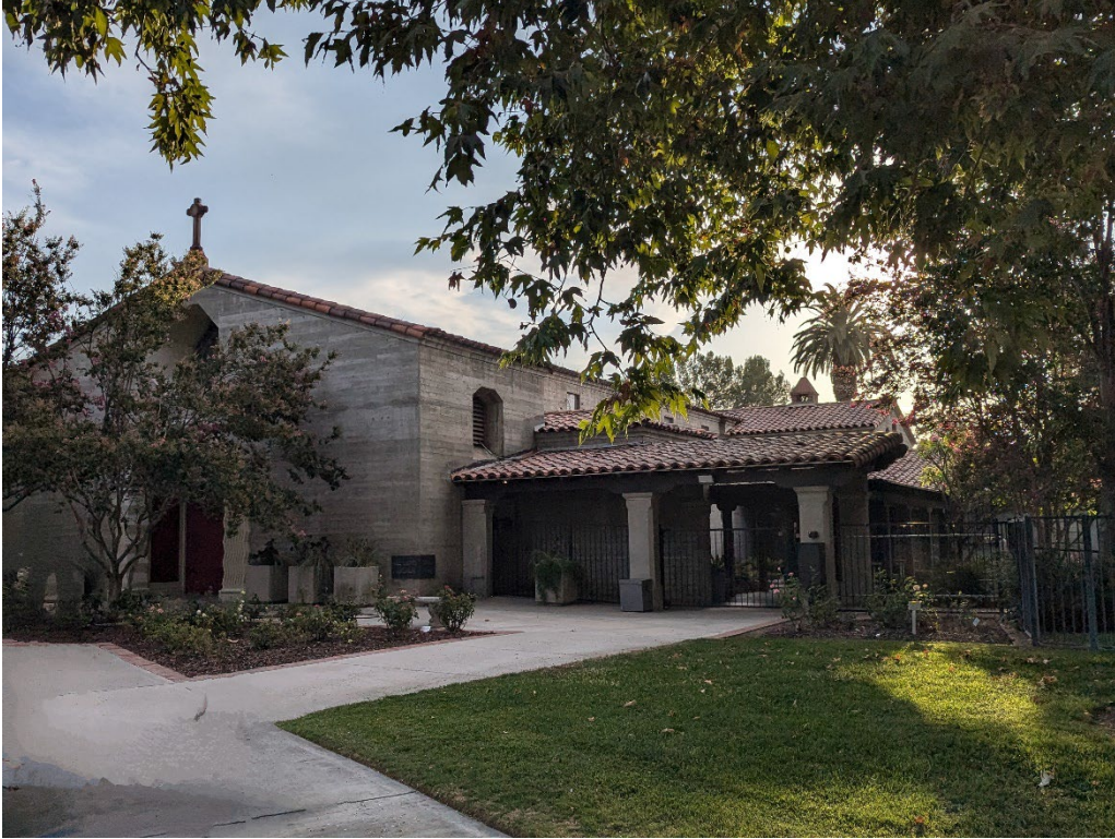
Figure 1 - Facade with arcade and pergola; view looking northeast
