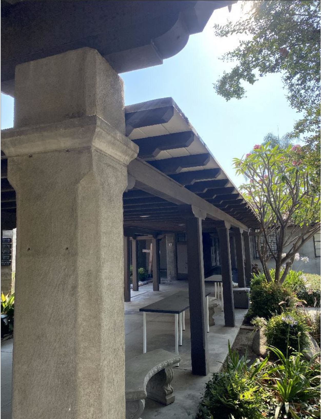
Figure 4 - Existing arcade post and pergolas
