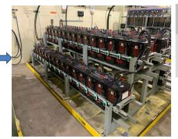
Typical Flooded Battery Bank (new standard)
