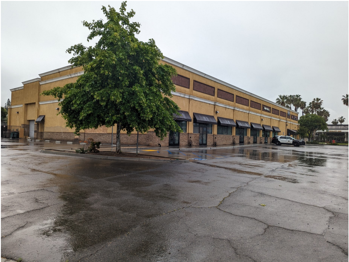
Southeasterly view of the existing building
