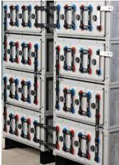
Typical Valve Regulated Battery Bank
