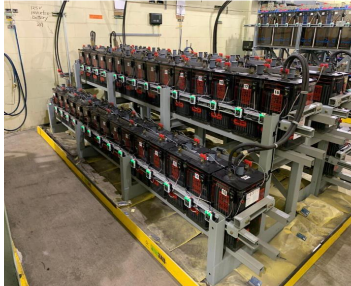
Typical Flooded Battery Bank
