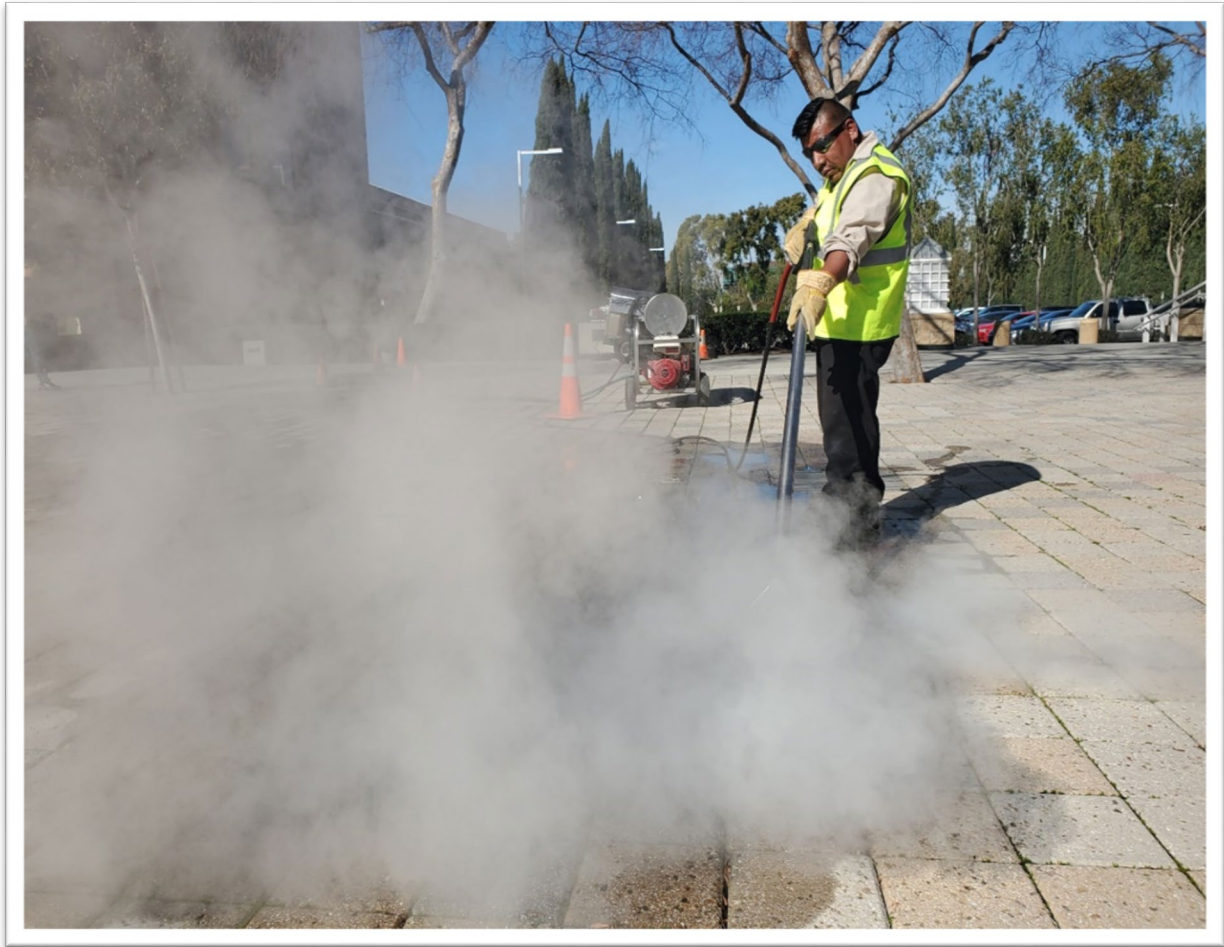
Example of a landscape contractor using steam to eradicate weeds in hardscapes.
